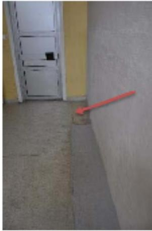
A photograph showing a dark-colored floor surface. A red arrow points to a small, irregular hole or tear in the material, indicating damage at the entrance of a room.                                                                    | <b>25 Dekker, gulv på grunn</b><br>Riss i ok gulv i WC gutter |
