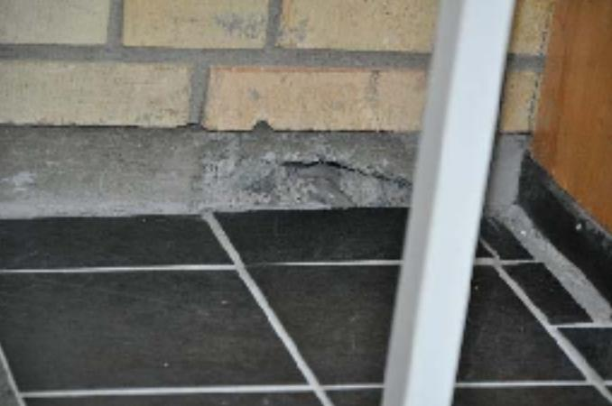
A close-up photograph of a concrete floor slab. A prominent vertical crack runs through the slab, starting from the bottom edge and extending upwards towards a white vertical pipe. The surrounding concrete appears aged and textured. | Avs kalling av betong i fm avløpsledning                      |
